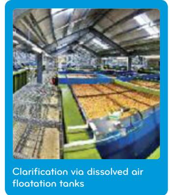
Clarification via dissolved air flotation tanks
