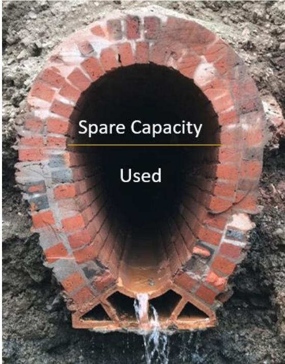
Figure 14 Brick Lined Sewer with the concept of Spare Capacity- Image courtesy of St John Archaeology
